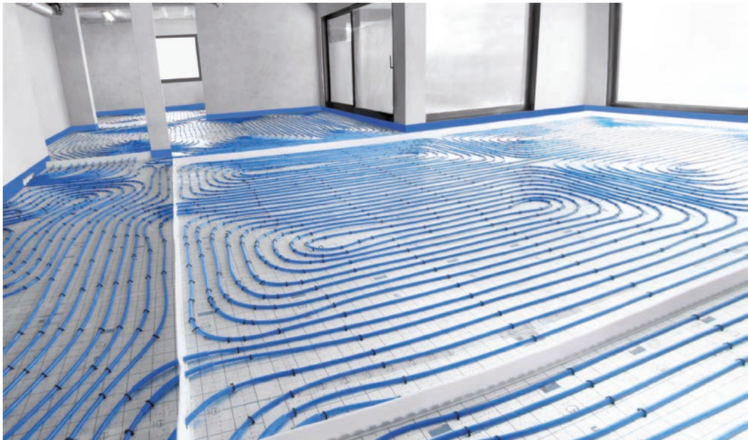
Fig. 24. KAN-therm Tacker System floor heating
