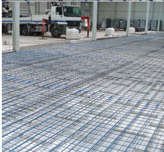
Fig. 4. Floor heating installation in industrial facility, employing PE-RT Blue Floor pipes and KAN-therm NET system.
