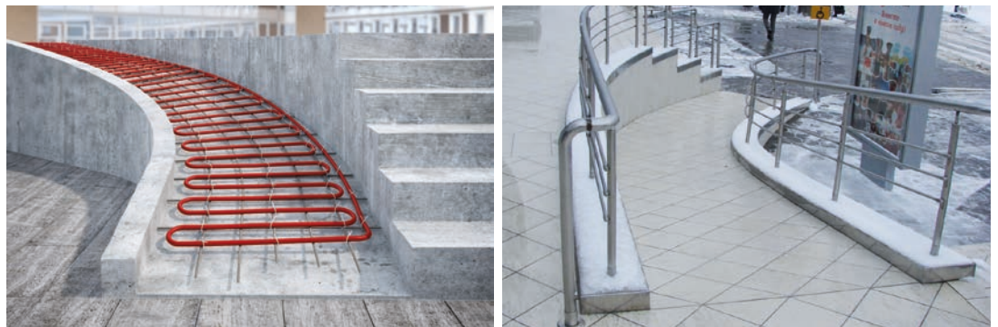
Fig. 41. KAN-therm External surfaces heating - during and after finishing of the works
