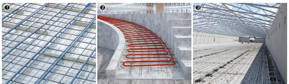
KAN-therm NET is a system of heating pipes mounting on various types of surfaces (on thermal insulation, on the ground, on concrete base). The design of surface heater (or cooler) may differ depending on the applied thermal insulation (or lack thereof) and on the type and thickness of layers over the pipes.
