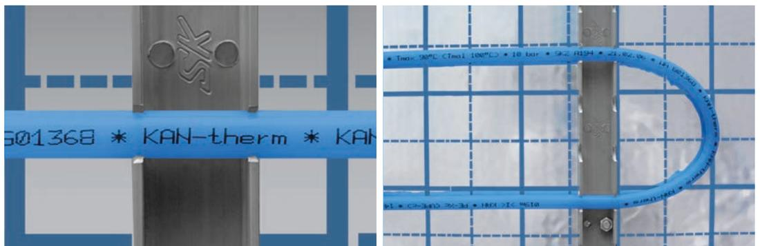
Heating pipes of 12 or 14 mm diameter are mounted on the wall in mounting strip, and then they are covered with a plaster layer of a total thickness of approx. 30-35 mm, forming a hotplate. The minimum plaster layer thickness over the pipe surface is 10 mm.
