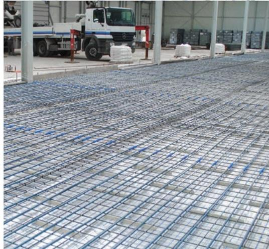
**Fig. 5.** Heating installation of outdoor patio employing KAN-therm system PE-RT pipes.
