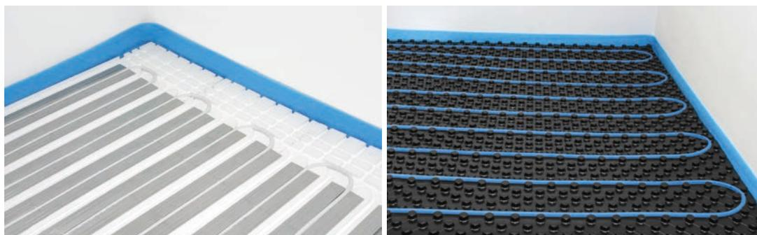
All heating plate contact points with vertical building partitions should be separated by a perimeter dilatation (spacing of at least 5 mm must be maintained). Dilatation should also be performed along the entire length of the doorway thresholds.
